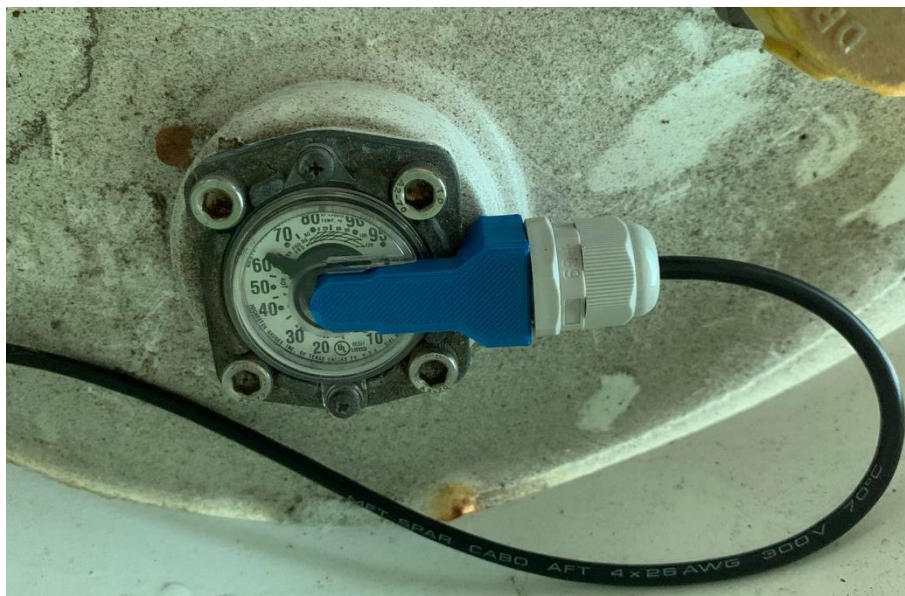
Figura 11 – Magnetron Drava com visor R3D e sensor i9GLP
